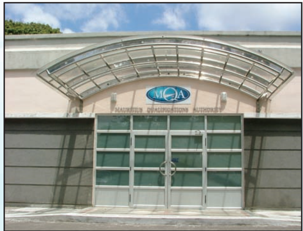
Main entrance of the MQA building
